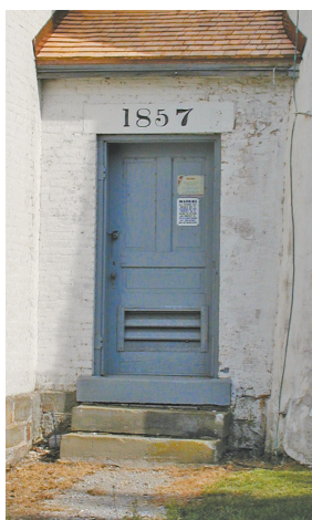
The lintel stone over the tower door with the 1857 build date.
