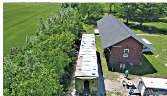
An overhead view of K102 and the Deckerville Depot while under restoration.
