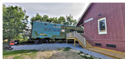
The K102 with its newly completed handicap accessible ramp and stairway.
