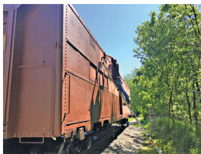
The exterior of the K102 gets primer applied by hired hand Ben.
