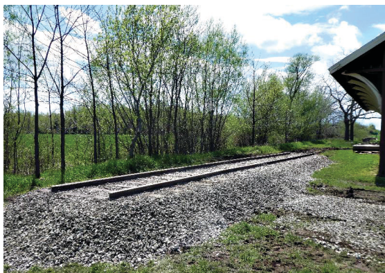
The finished panel track awaits the arrival of the Troop Kitchen Car.
